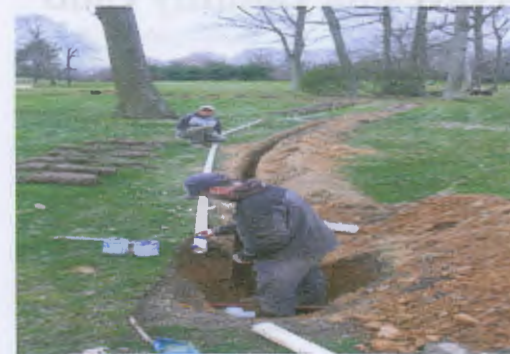
Irrigation installation in the fall / winter
