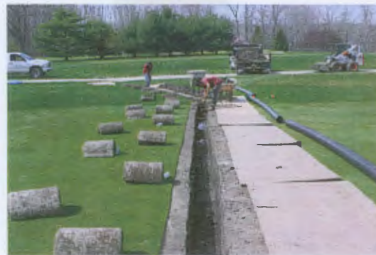
Ongoing drainage projects.
